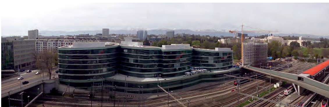
View of the Maison de la Paix with Tower 5 under construction
